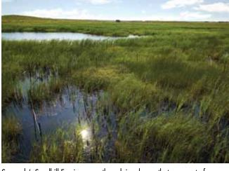
Syncrude's Sandhill Fen is a recently reclaimed area that was part of a now-depleted oil sands mine. It was built on a foundation of mine tailings called composite tails.
